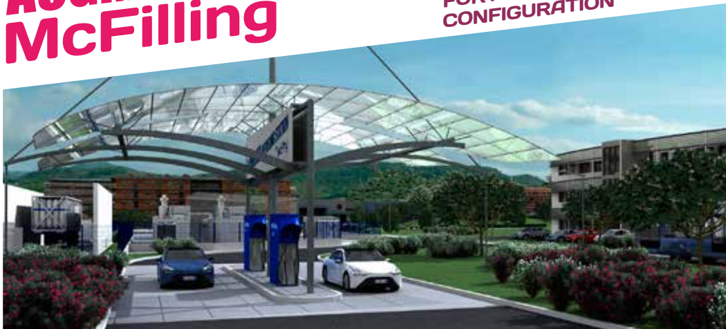
Hydrogen Recharge Infrastructure ("HRI") 1,600 kg / day configuration, including a McLyzer 800-30 for on-site production of the equivalent of 4 MW of hydrogen. Possible refueling scenarios: 320 light vehicles, 40 trucks, 80 buses, and possibility of exporting hydrogen by tube trailers up to 500 bar, for uses far from the production point.
