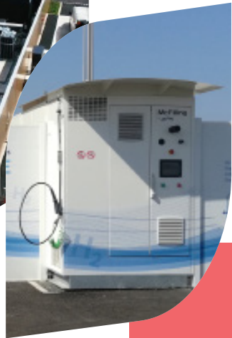
[ABOVE] In Béthune, 1 st zero-carbon hydrogen station for buses in France 200 kg / day | 0.5 MW electrolysis
