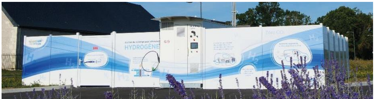
McFilling 20-350 hydrogen station in Sorigny
