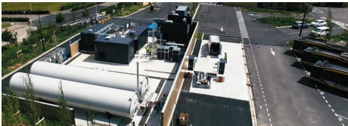
Haut de France, “SMT- AG” project: first zero-carbon hydrogen station for buses in France (200 kg of hydrogen / day, 0.5 MW electrolysis).
