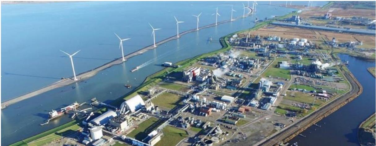
DJEWELS | On a chemicals plant in Delfzijl, Netherlands: McPhy was elected to install the largest industrial zero-carbon hydrogen production unit in Europe. 20 MW, 3,000 tonnes of zero-carbon H 2 / year, 27,000 t.CO 2 avoided / year 6
