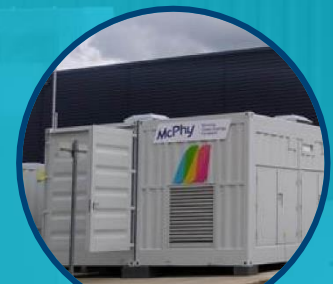
APEX Energy Installation of a 2 MW electrolyzer in Germany
