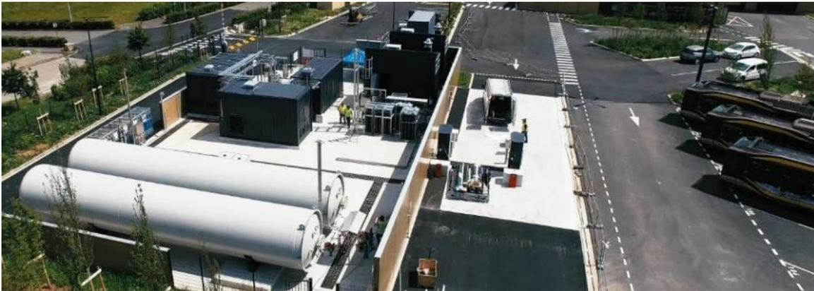
Haut de France: first zero-carbon hydrogen station for buses in France (200 kg of hydrogen / day, 0.5 MW electrolysis).
