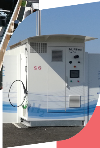
[ABOVE] In Béthune, 1 st zero-carbon hydrogen station for buses in France 200 kg / day | 0.5 MW electrolysis
