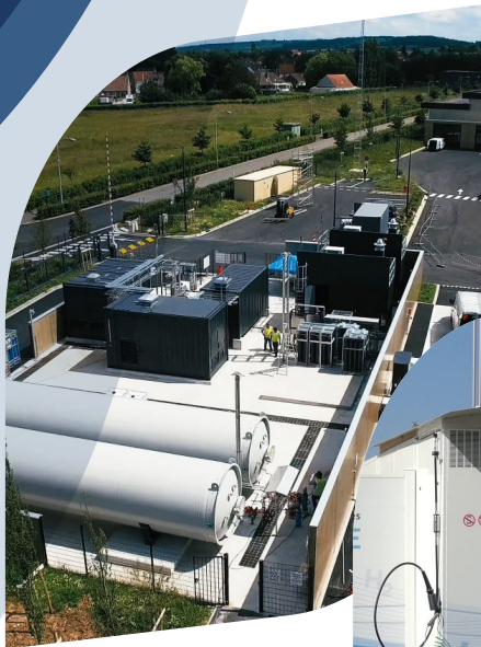
[ABOVE] In Béthune, 1 st zero-carbon hydrogen station for buses in France 200 kg / day | 0.5 MW electrolysis
