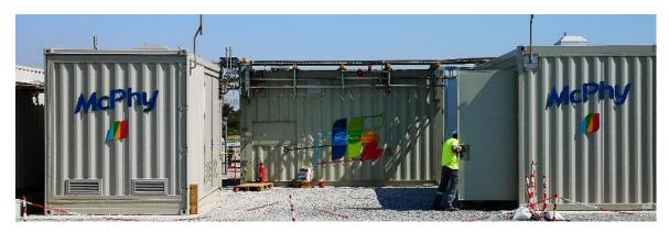
Jupiter 1000: 1 MW of electrolysis for a PtoG demonstrator in Fos sur Mer (0.5 MW alkaline + 0.5 MW PEM)
