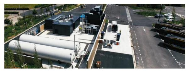
Haut de France: first zero-carbon hydrogen station for buses in France (200 kg of hydrogen / day, 0.5 MW electrolysis).
