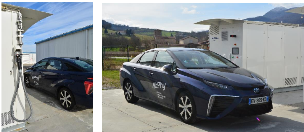
Illustration of a McFilling 20-350 station equipped with an infrared connector for partially refueling 700 bar vehicles (Toyota Mirai pictured). A large number of car manufacturers are committed to hydrogen and an increasing number of 700 bar models is available for sale.
